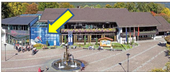
Conference Center building
