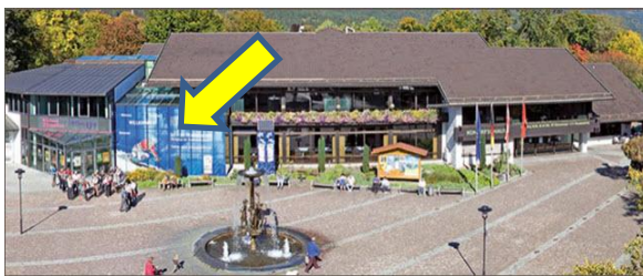
Conference Center building
